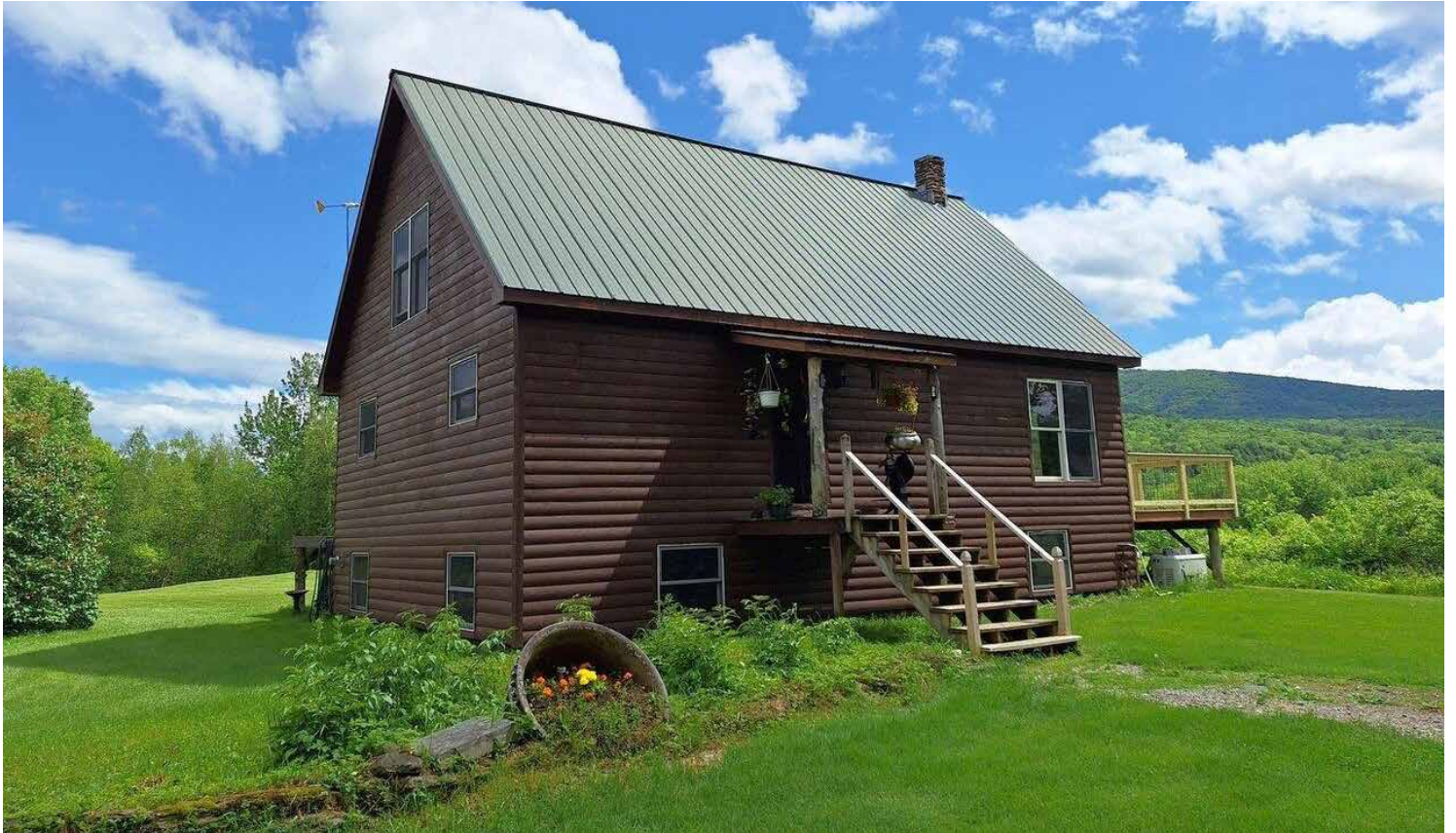
2728 VT Rte 109, Cambridge, VT ~ An amazing off-grid opportunity awaits new owners of this beautiful solar powered, 2-bed, 1-bath home with stunning river & mountain views, woods, & large, private, sandy river beach.
